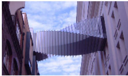
The Bridge of Aspiration connects London's Royal Opera House with the Royal Ballet School.
